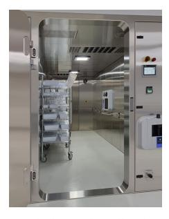
PBSC's chambers were designed bespoke to Hikma's requirements, being the longest chambers at 6m long PBSC has produced for MDS to date. Integrated into Hikma's cleanroom environment for the purpose of decontamination of material/equipment transfer.
